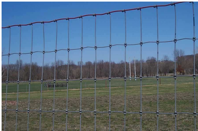
Photo 2 2"x4" grid "No Climb" woven wire fencing. Used in small dog yard, training yard, and entrance area.
