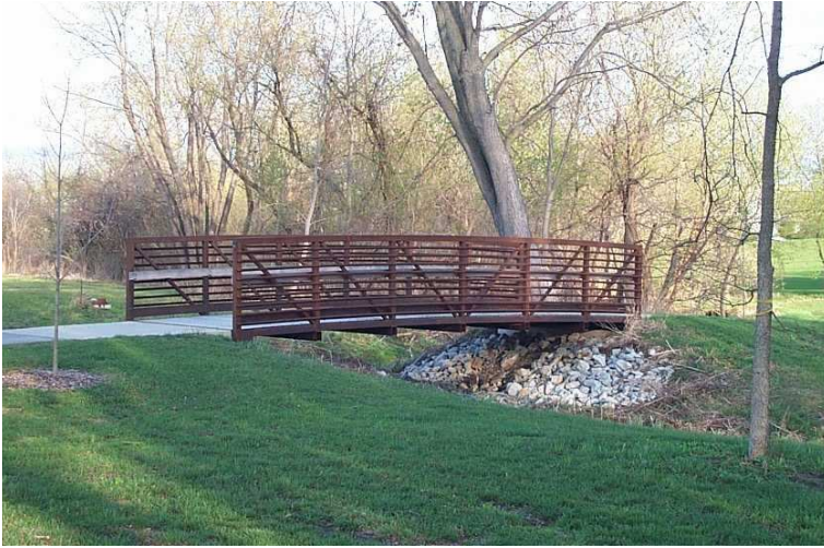
Photo 1 Bridge at Hunter's Run Park
